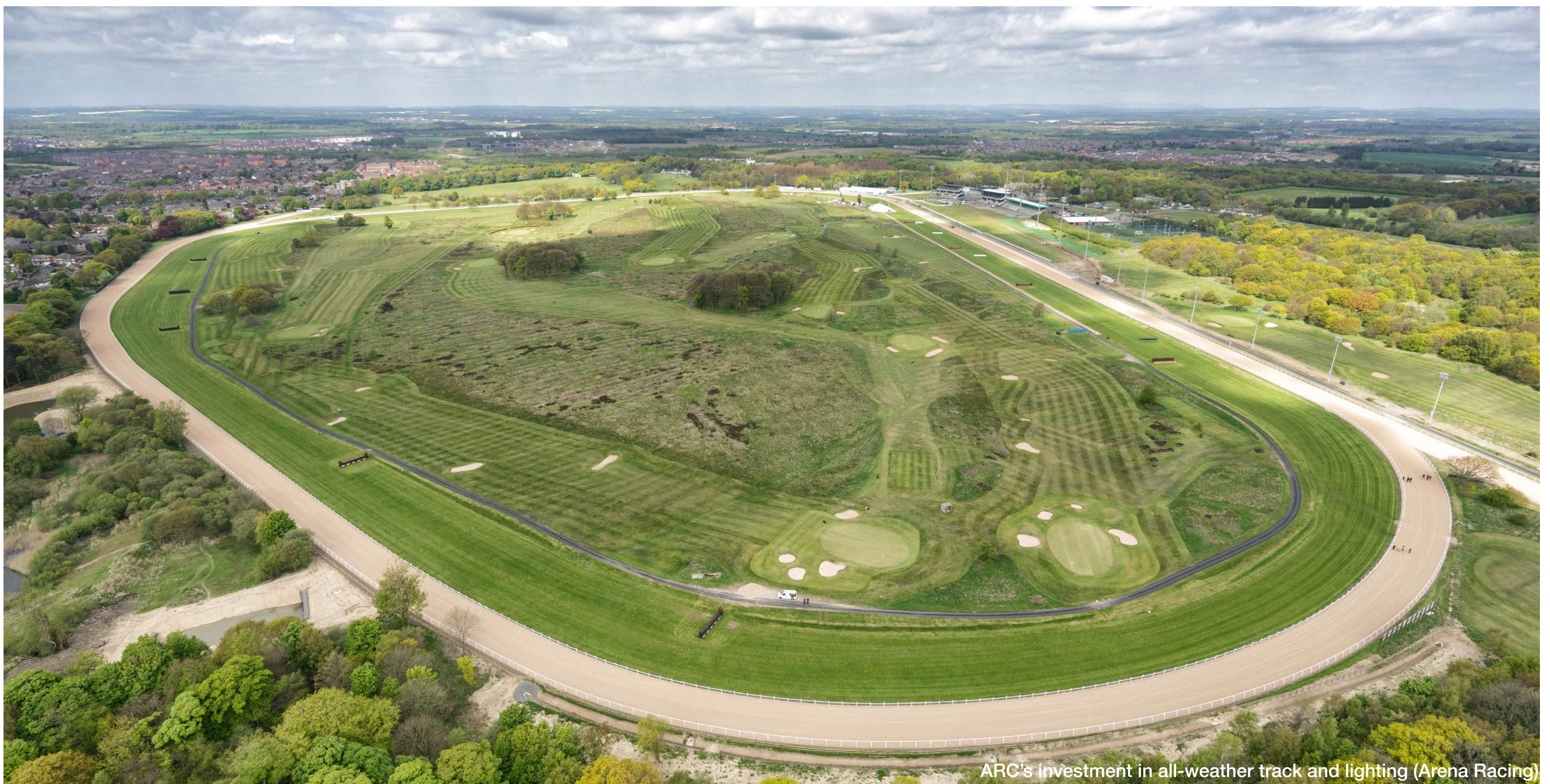
Forthcoming refurbishment of stands
